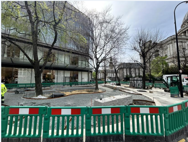
Cheapside Sunken garden progress, due to be completed in May 2024.
